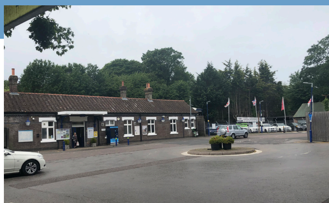
Existing view north-west towards train station.
